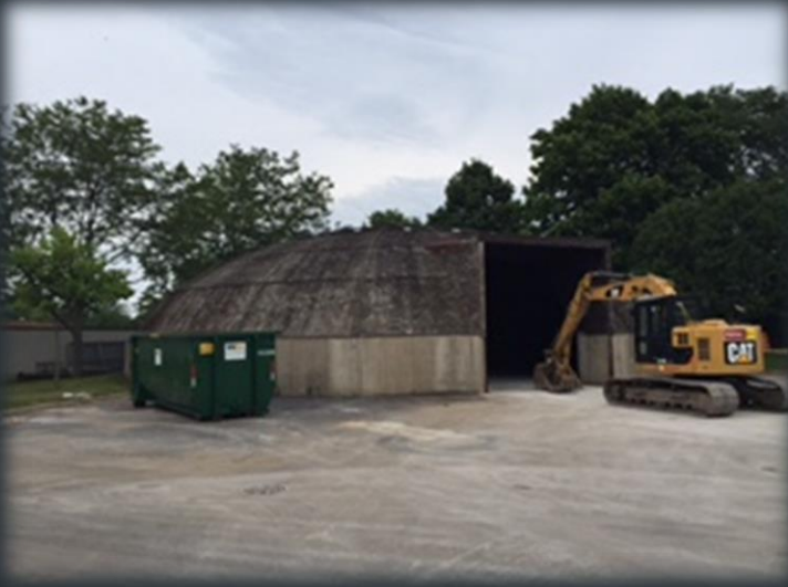
Old Salt Storage Facility – 1,850 Ton Capacity
