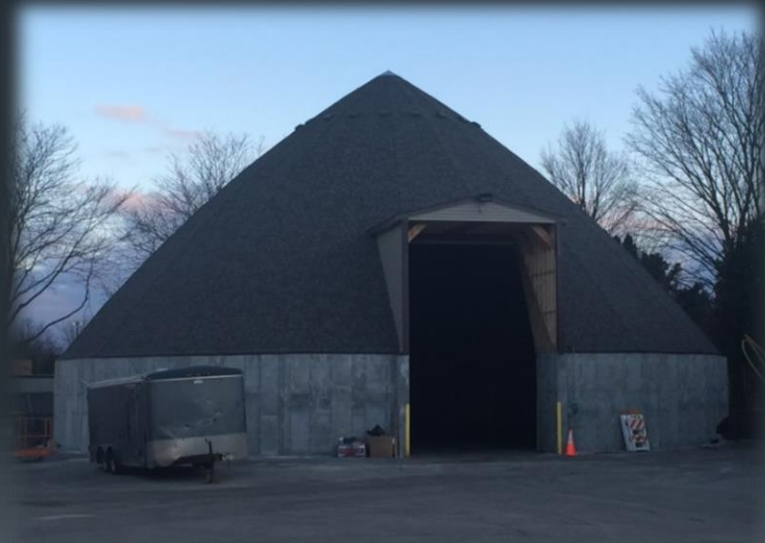
New Salt Storage Facility – 3,700 Ton Capacity
